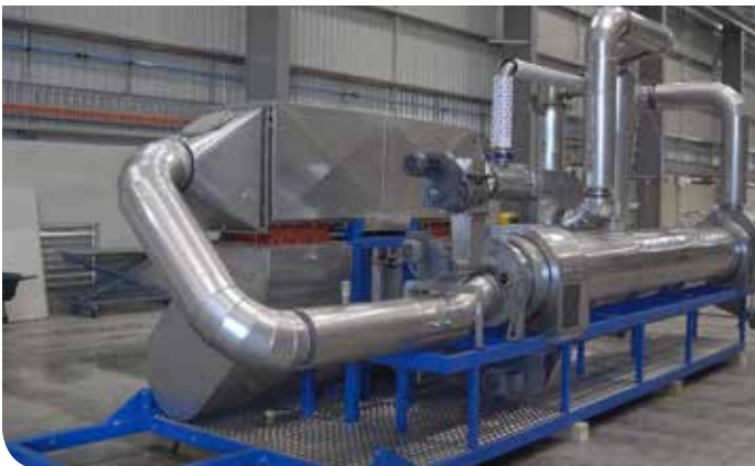
Airless Dryer testing unit with an evaporation rate of 125 kg/hour (275 lbs/hour)
